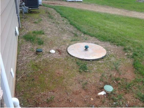
Photo above-Grinder pump station with fiberglass tank and stainless steel lid installed outside a home
